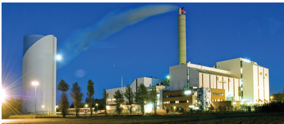
Ilustrační foto: Nyköping combined heat and power plant by Vattenfall @Flickr.com
